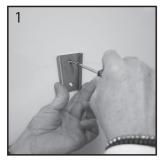
Attach the Tube with the included mounting hardware at 1,2 meters of max. height.
